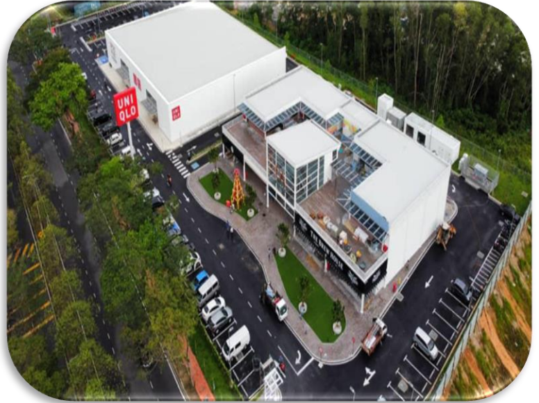
UNIQLO TOMBO Rock Mineral Wool used for Roof Insulation
